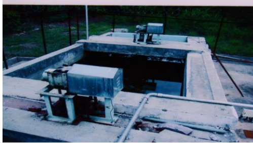
Fig.3.1 Surface Aerators in the Aeration Tank
