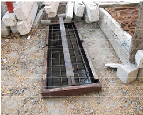
Figure-2: casting of Steel and concrete composite beam without steel encased
