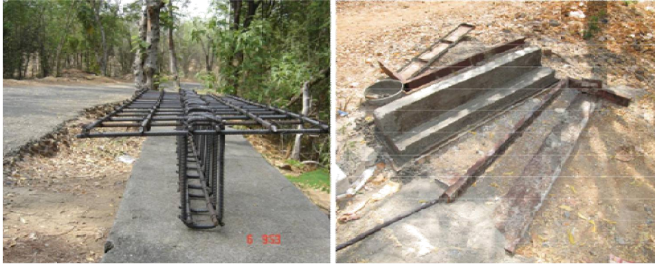
Figure-1: Casting of RCC beam
