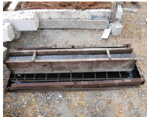
Figure-3: casting of Steel and concrete composite beam with steel encased
