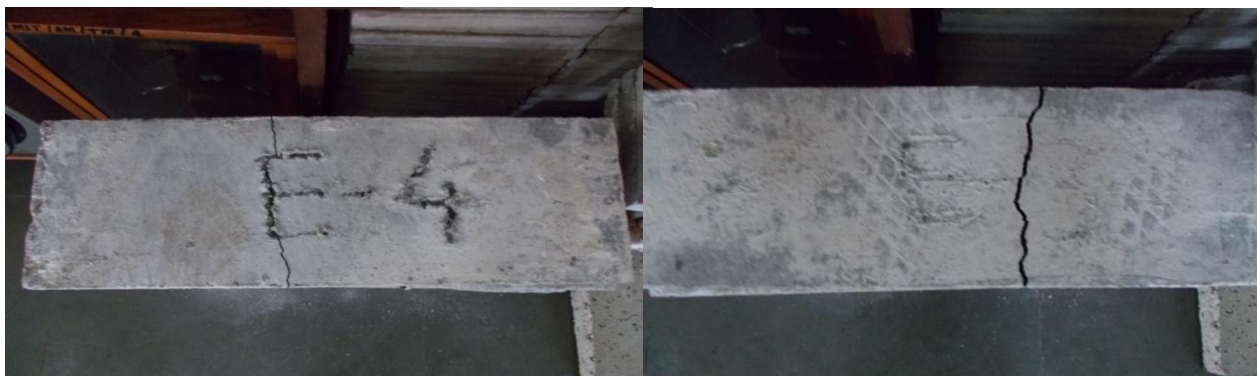
Fig. 12. Typical Top view of crack pattern for 40mm and 50 mm thick panel
