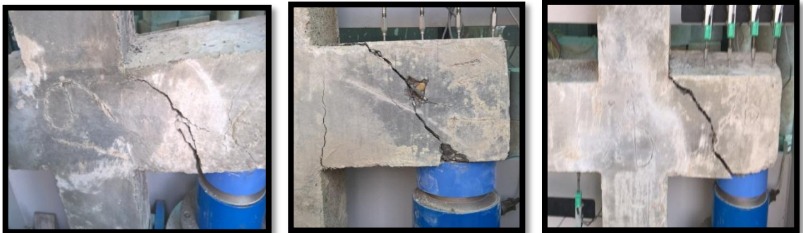
Fig.9(i) RC Joint 6% Fibre Cracks (ii) RC Joint 9% Fibre Cracks (iii) RC Joint 12% Fibre Cracks
