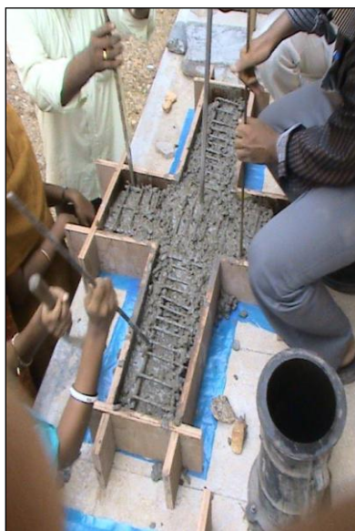
Fig.2: Casting of beam column joint
