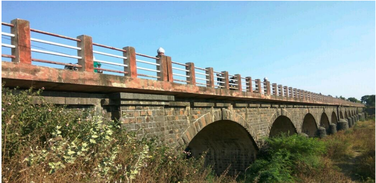
Fig 4: Photograph of Pedhi river bridge site
