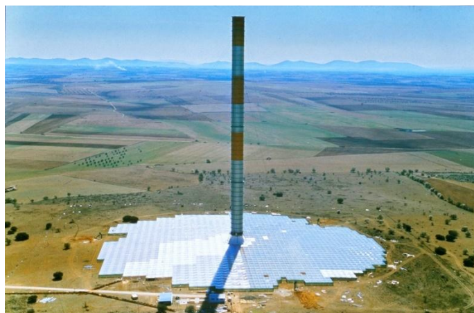
Fig..2The firstSpanish prototype that was built in 1982 before collapsing in 1989
