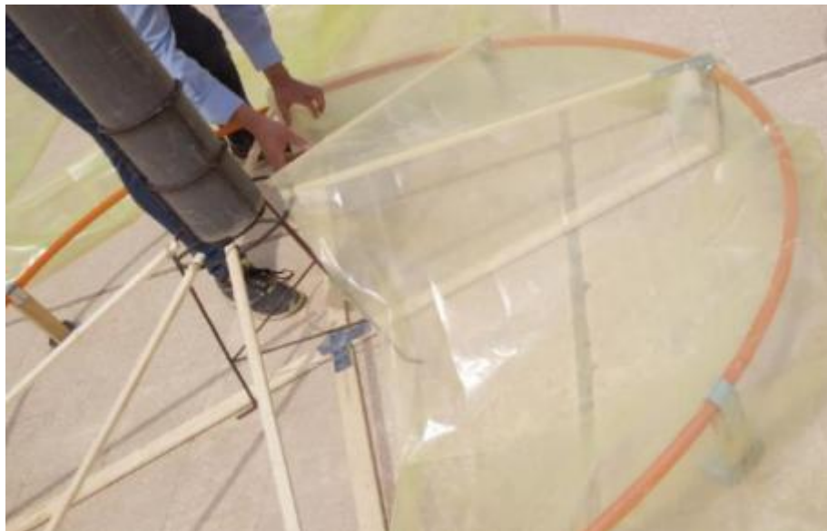
Fig..10The final step in covering the solar base with polyethylene
