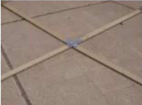
Fig.6 the cross shape formed by 4 wooden pieces connected by aluminum extension
