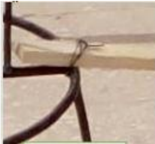
Fig.8 wood pieces are connecting the metal base with the rounded PVC tubes. Fig..96 wood pieces are connecting the metal base with the rounded
