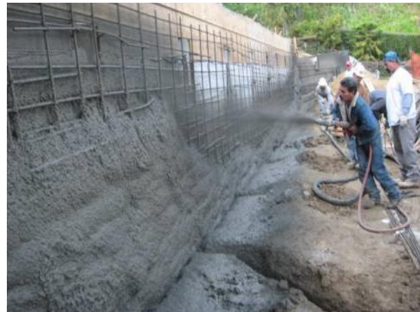
Figure No. 12 Application of shotcrete over RCC Retaining wall Surface
