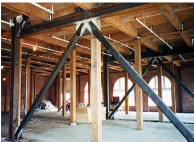
Figure No. 15 Application of Steel Bracings
