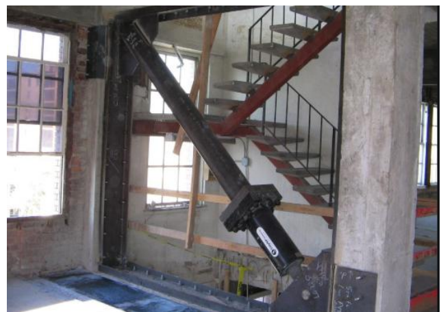
Figure No. 15 Application of Steel Bracings
