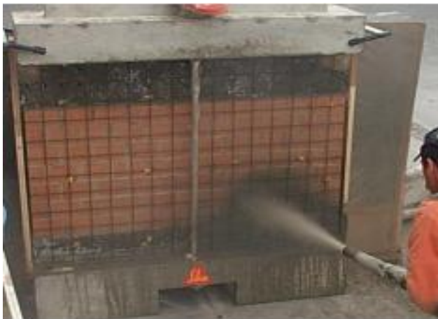
Figure No. 11 Application of shotcrete over Masonry surface
