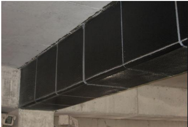
Figure No. 3 Carbon FRP fibre installation and Composite Strengthening services
