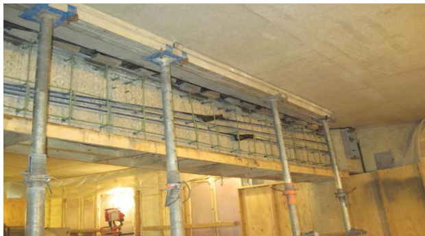
Figure No. 1 External Post Tensioning
