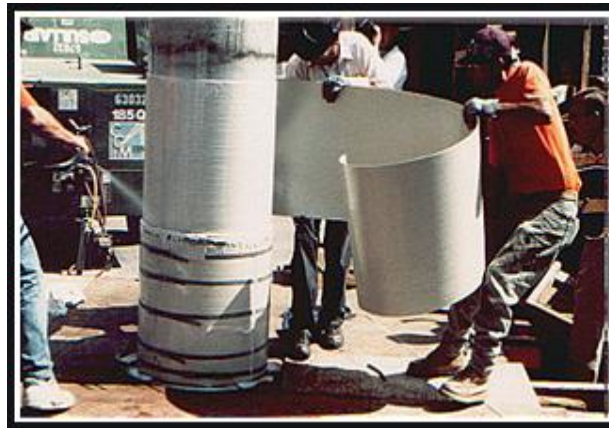
Figure No. 14 Installing Prefabricated Fiberglass jacket
