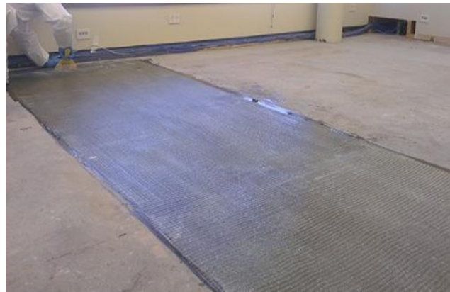
Figure No. 4 FRP composite Strengthening with Concrete solutions
