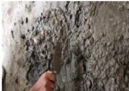
Fig.No(9)preparation of concrete
