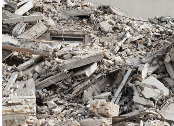
Fig.3 Waste from Demolition of building
