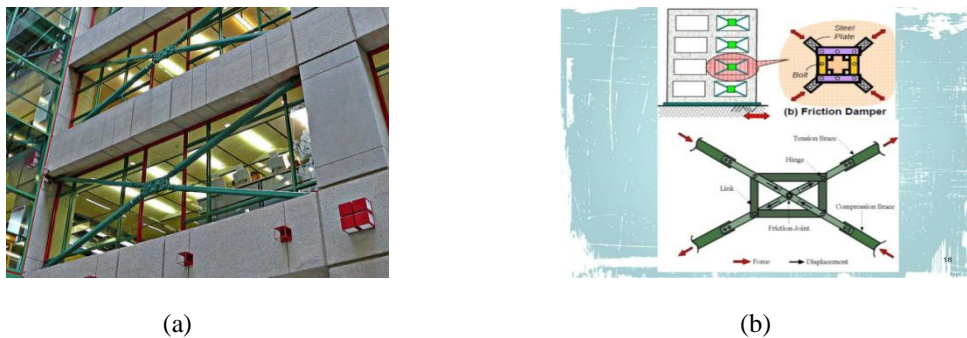
Fig. 2.1.1- Friction Damper.(a) Webster Library of Concordia University in Montreal, Canada.(b) represent the system design of this system.
