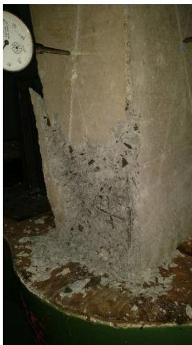
Fig8: CRC1a Column Failure
