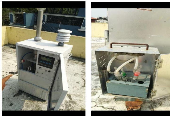
Fig. 2. Manual monitoring machines at Vytilla, Ernakulam , Kerala
