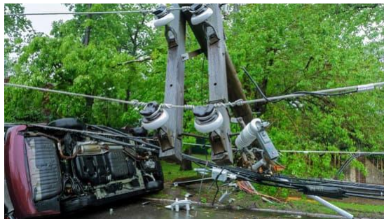
Figure 1: Damaged pole under dangerous situation.
