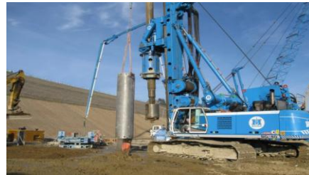
Fig 6. Kelly drilling
