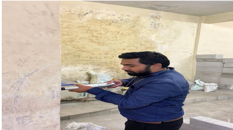
Picture 1: Rebound Hammer NDT Testing on Column
