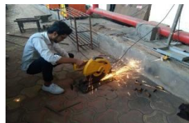
Figure 2.4. Making of steel mesh
