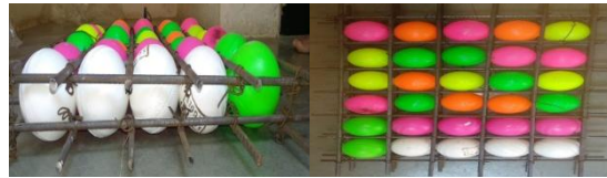
Figure 2.5. Bubble deck slab mesh
