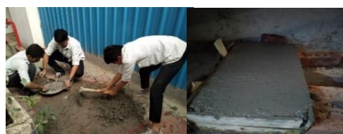
Figure 2.2. Mixing of concrete and casting of slab
