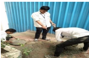
Figure 2.7. Preparation of concrete
