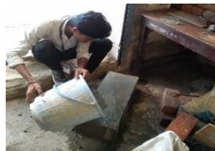
Figure 2.8. Curing of concrete Slab
