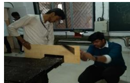
Figure 2.6. Preparation of formwork
