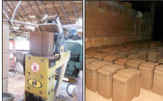
Fig3. Casing of Interlocking Mud Blocks through Hydro form Machine in Field:
