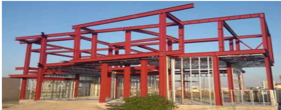
Fig No 2 Conventional steel Building.
