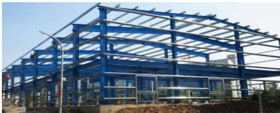
Fig No 1 Pre-Engineered Building (3D)
