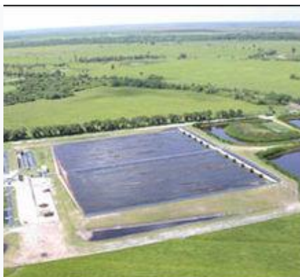
2.5 acre ATS system, installed by Hydromentia on a farm creek in Florida
