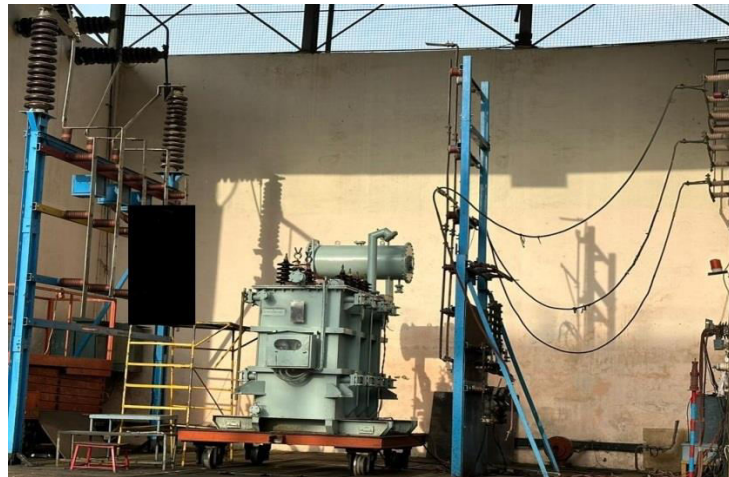
Fig. 5 Power transformer under short circuit test in CPRI, STDS, Bhopal.
