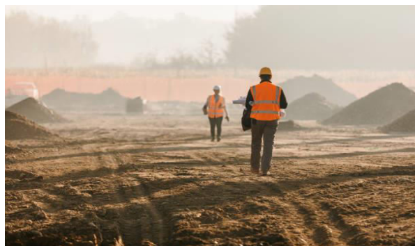
Fig.5 Construction workers evaluating work at site for soil testing
