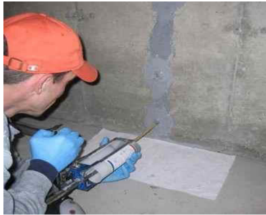
Figure 2: Epoxy Injection
