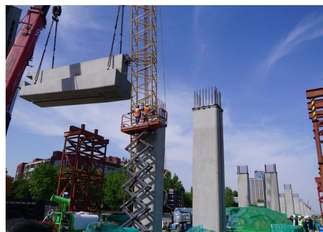
Fig. 3 The green construction technology—prefabricated bridge construction (a) The standardized centralized prefabrication of components in the precast factory (b) The on-site hoisting, installation, and connection of prefabricated components
