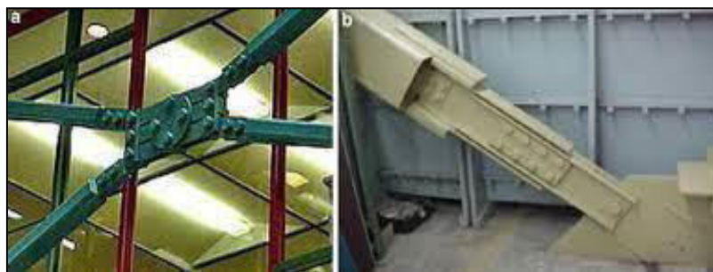
Figure 2: Friction Damper
