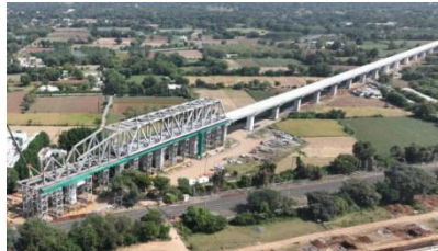
Fig 1:- Image of truss bridge Mumbai-Ahmedabad High Speed Rail Corridor
