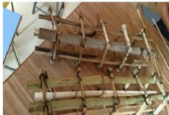
Fig. 9. Reinforcement of Beam
