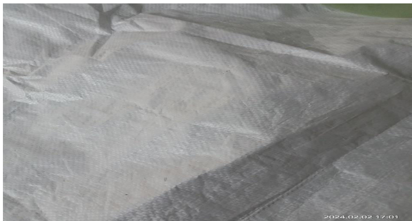
Fig.11 Plaster used in curing pad to prevent water from evaporation.
