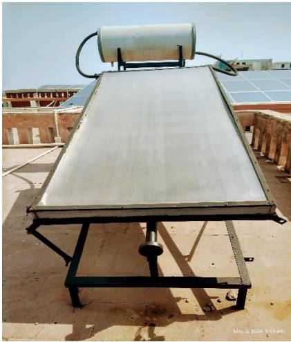
Fig: Schematic Diagram of solar flat plate collector
