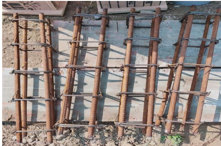
Fig :- Reinforcement bars
