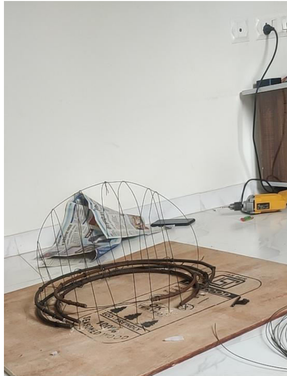
Figure.1- construction of foundation
