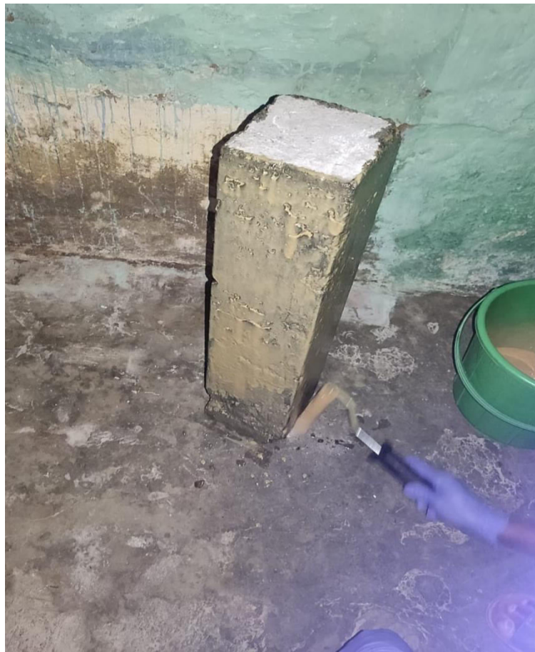
Fig :- Application of Resin
