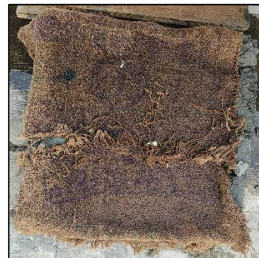
Figure 3: Conventional Slab Curing
