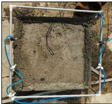
Figure 2: Sensor Based Slab Curing
