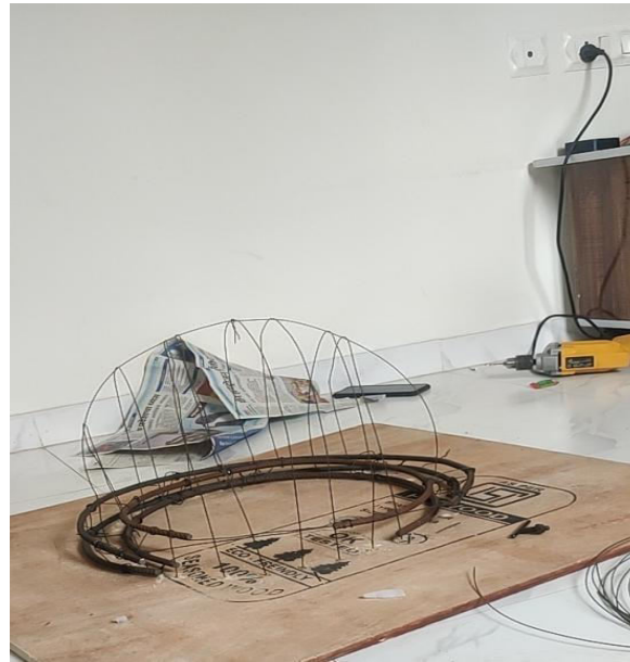
Figure.1- construction of foundation
