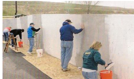
Fig.5 Painting of Structure
