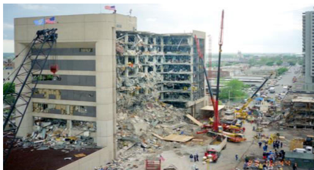
a) Alfred P. Murrah Federal Building Collapse
