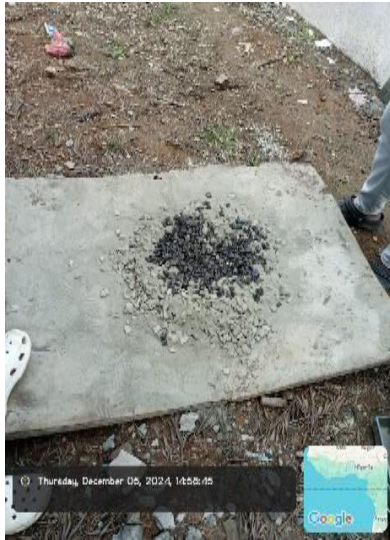
a) Preparation of concrete mix
