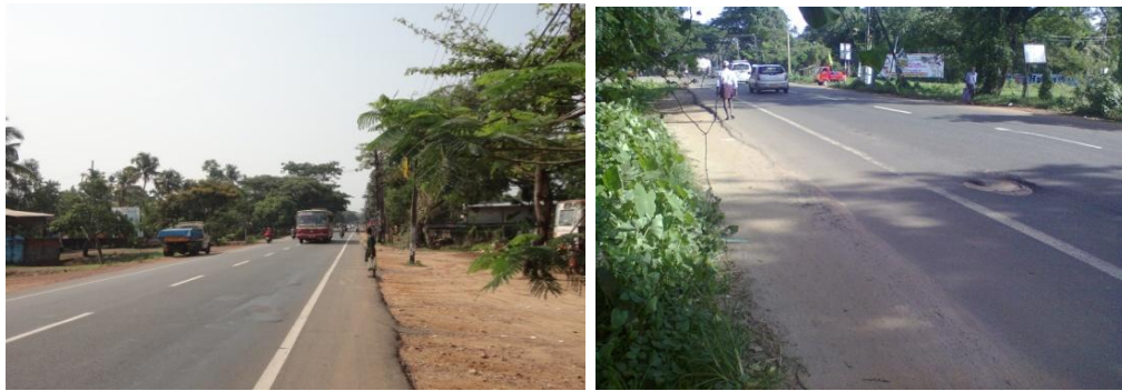
Fig 3: Kalavoor accident location
